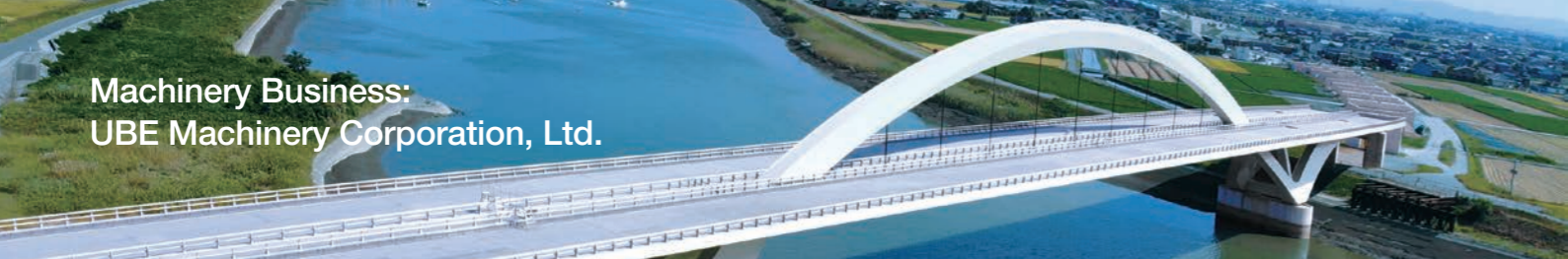
Hayatsue River Bridge
