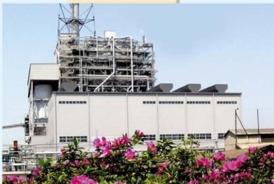
IPP power plant
