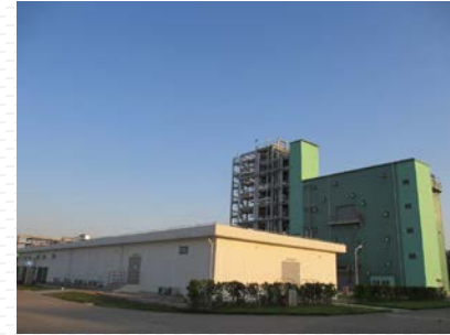
Electrolyte manufacturing at Advanced Electrolyte Technologies (Zhangjiagang)
