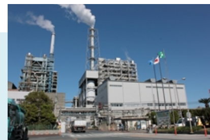
IPP power plant
