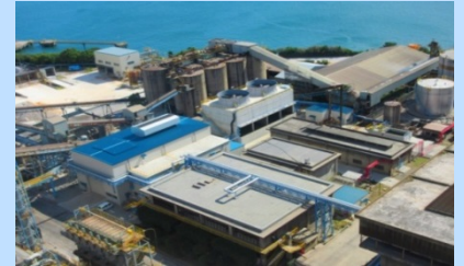
Exhaust heat recovery system
