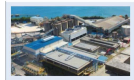
Exhaust heat recovery power plant
