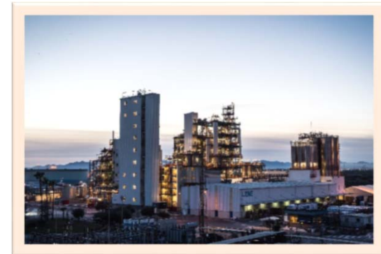
New nylon plant in Spain
