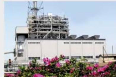
IPP power plant
