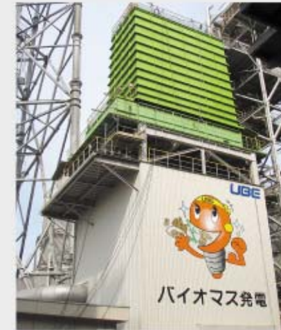
Biomass fuel facility
