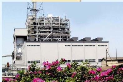
IPP power plant
