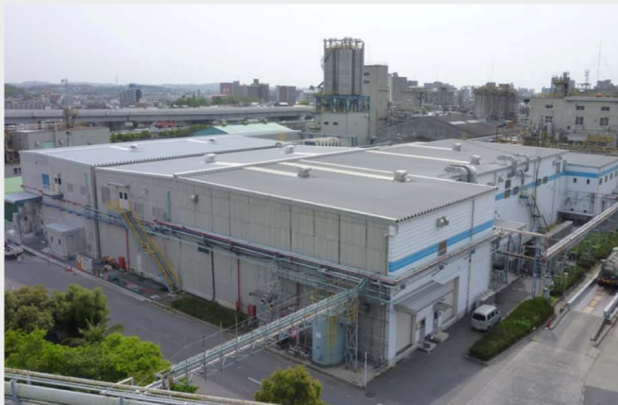
7th production facilities for separator films (Ube, Yamaguchi)
