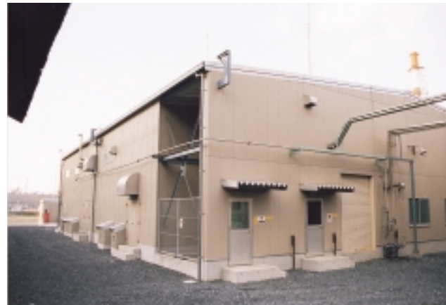
■ Metal organic (MO) compounds manufacturing facility
