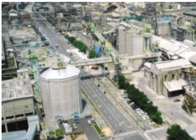
■ The eastern wing of the UBE Cement Factory, which has recently been modernized
