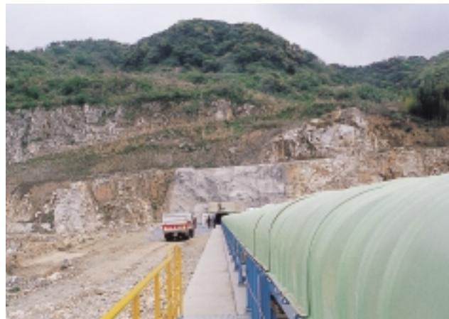
■ Limestone transportation facility at the Kanda Cement Factory (a joint project with Mitsubishi Materials)
