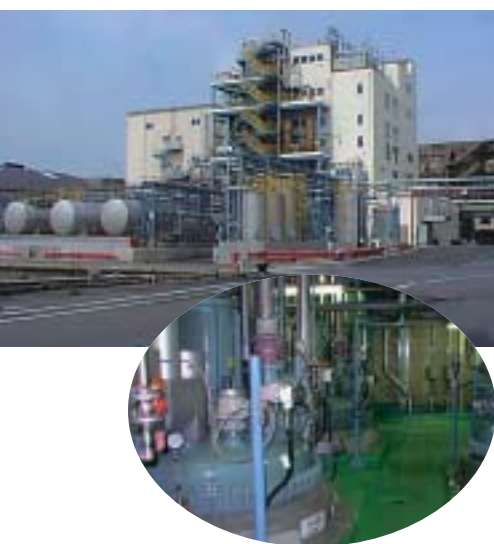
Ube Industries' second pharmaceutical products manufacturing plant (exterior and interior)
