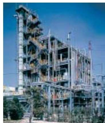
EUP's pressurized two-stage gasification process facility
