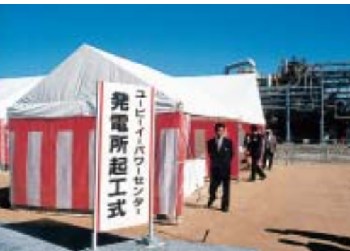
Inauguration of the UBE Power Center's power generation plant
