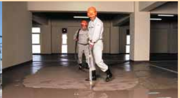
Application of self-leveling materials
