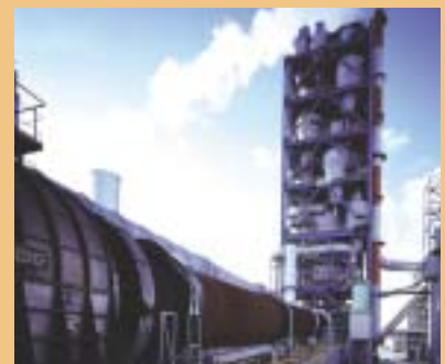
The new suspension preheater kiln at the Ube Cement Factory
