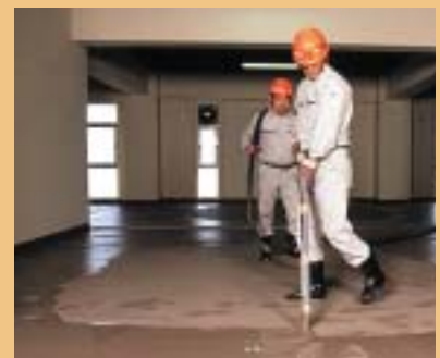
Application of self-leveling materials
