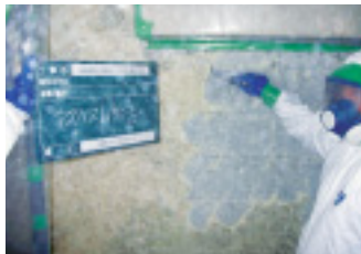
Removing asbestos
