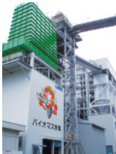
216 MW pulverized coal/thermal power/biomass fuel manufacturing facility
